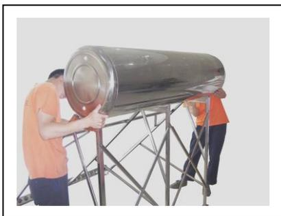
Put the water tank on the bracket
