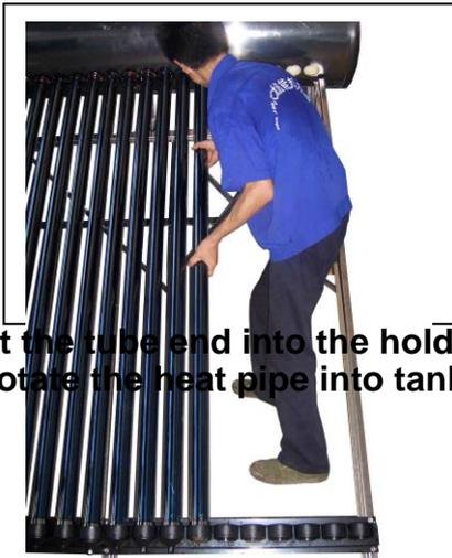
**Insert the tube end into the holder, then rotate the heat pipe into tank slowly**
